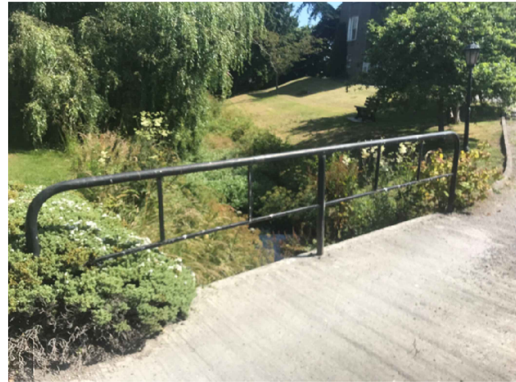
Existing bridge to Parochial House to be railed for safety
