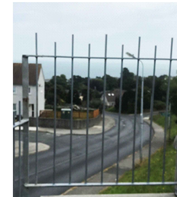
Simple galvanised metal railing edge protection
